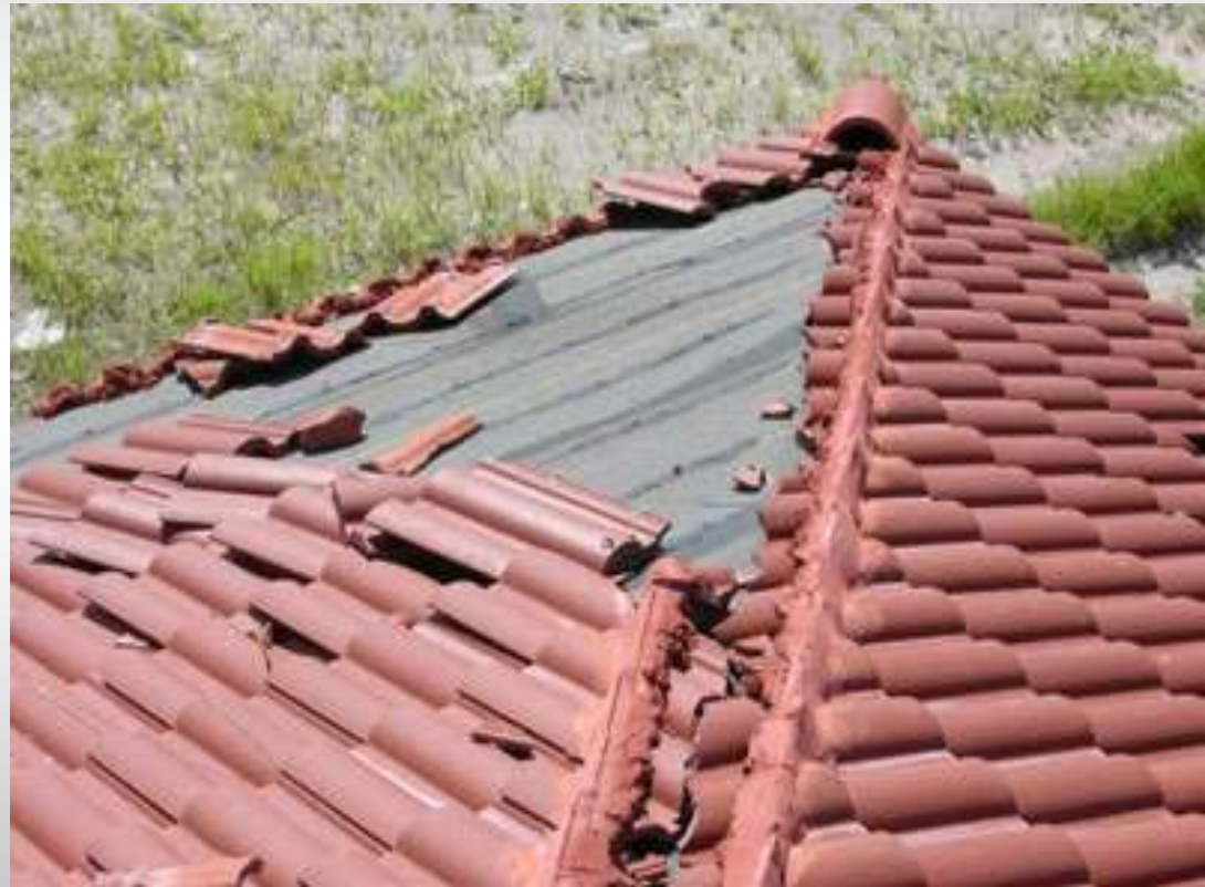
Hurricane (typhoon) damage
